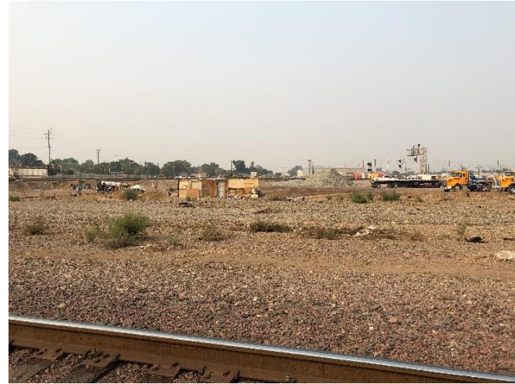
Representative Project Photos (Rail Crossing): None, looking west (37.94699592742171, -121.27223642223692)
